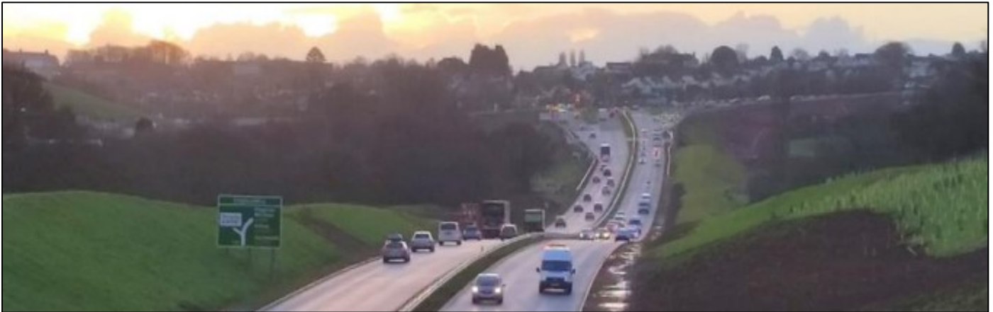
Figure 17: South Devon Link Road completed scheme
