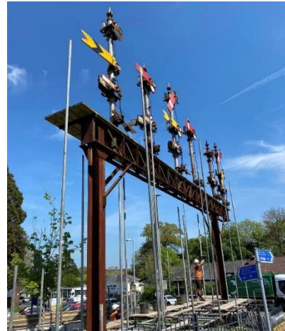
Scaffolding going up May 2024
